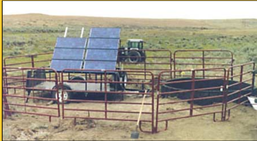
A trailer-mounted PV system is improving range management and water quality along Painted Robe Creek near Lavina, MT.
