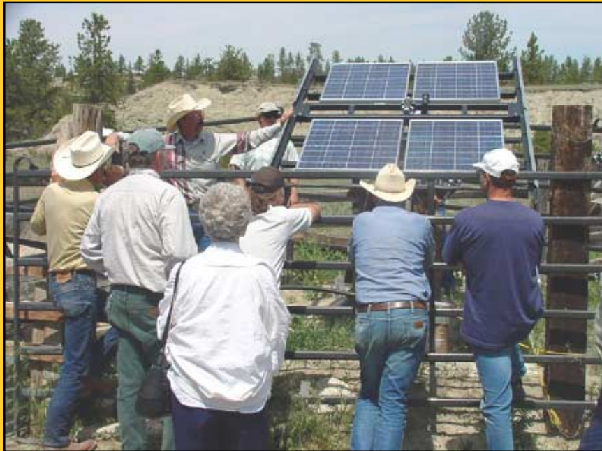
A tracking PV array replaced an old and unreliable windmill on the Ballard Ranch near Lavina, MT.
