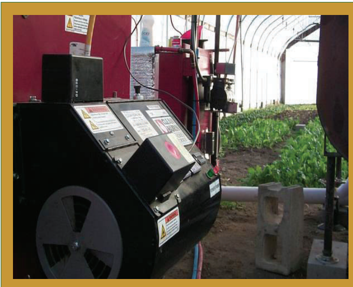
Laughing Stock Farm's waste restaurant oil burner heats the farm's winter greenhouse.
