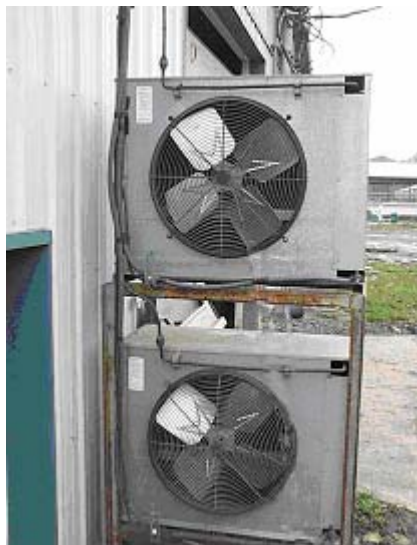
Figure 2-4. Example of a remote air-cooled condenser
